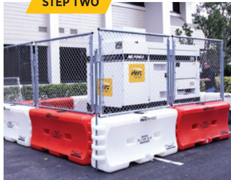
Fence and crash barrier
